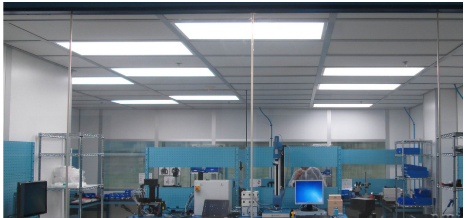
Cleanroom Production in Auburn, USA (Photo: VolpiUSA)
